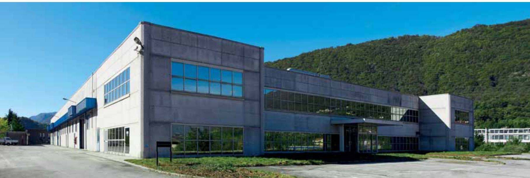
New building opening August 2018
